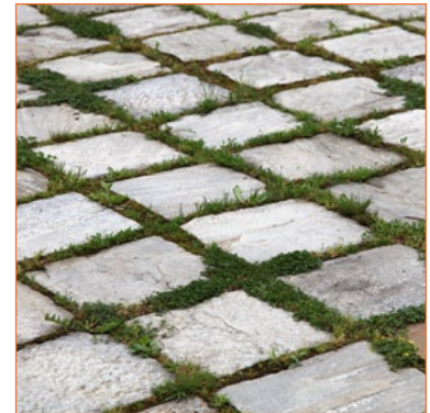
Example of laying sets in stack bond pattern using grass cross spacers
