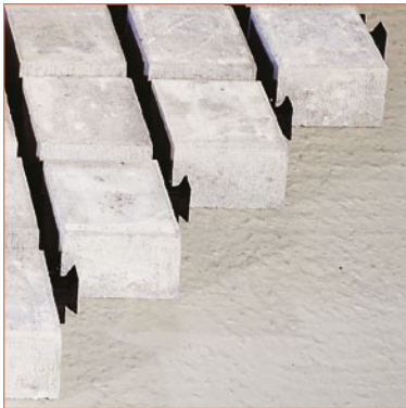
Laying grass cross spacers
