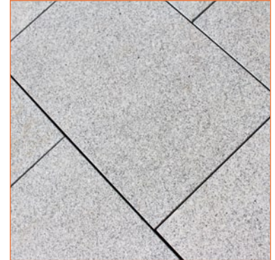
Example of laying in a running bond pattern
