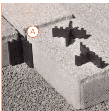
Laying T-shape spacers
