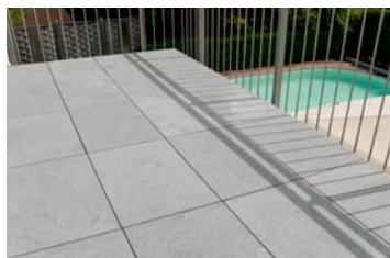
... the slabs are always laid at right angles and truly aligned. This gives you a stable surface and an even pattern of joints.
