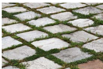
Example of laying setts in stack bondpattern using GRASS CROSS SPACERS
